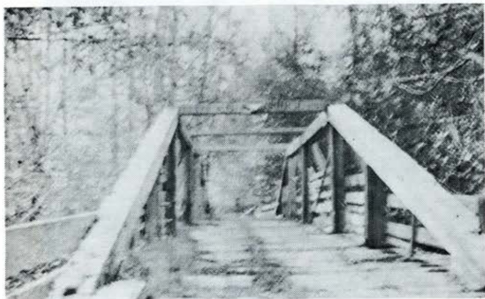
Elkhorn Bridge -- West Millicoma River 72 Foot Span -- 1896 Built by George Gould and Sons using 2 Yoke of Oxen Hewn Red Cedar Timbers Sawed Planks for Decking
