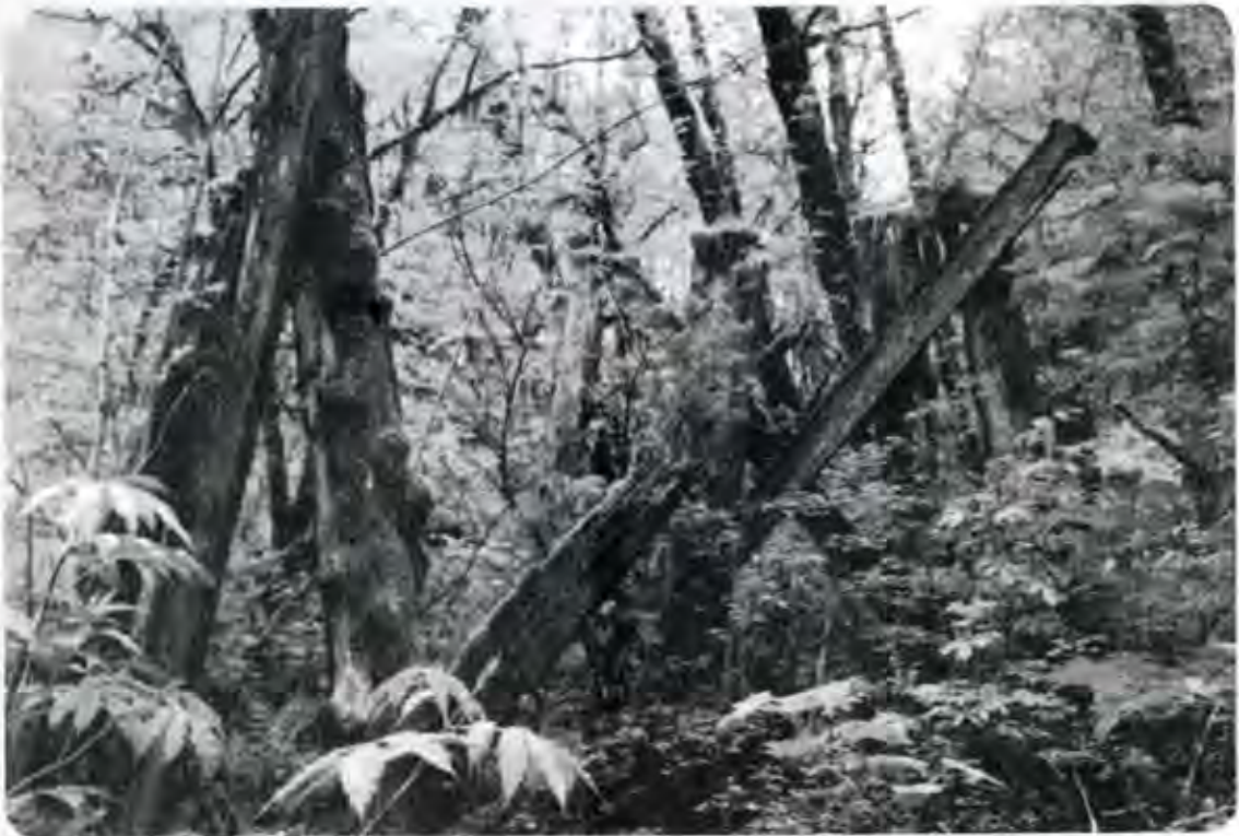
Rotted remains of 1930 logging railroad trestle on Marlow Creek. —Photo by Author, about 1960.
