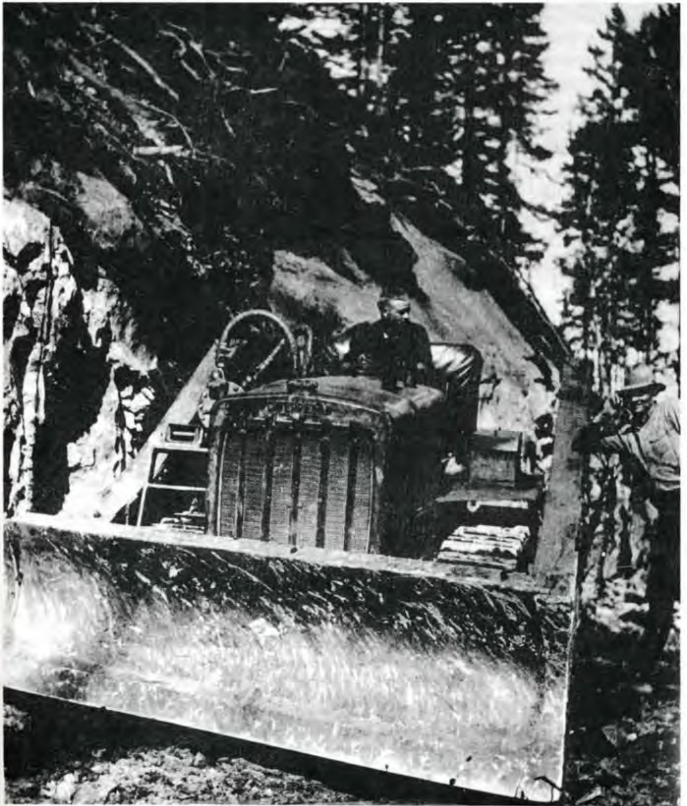
One of the Camp Walker "gas 50" cats working on Scholfield-Umpcoos construction (1935). The CCC tractors didn't have canopies or other protection for the men who operated them. The small number of injuries seems truly amazing to me. — Photo courtesy Coos Forest Protection Association files.
