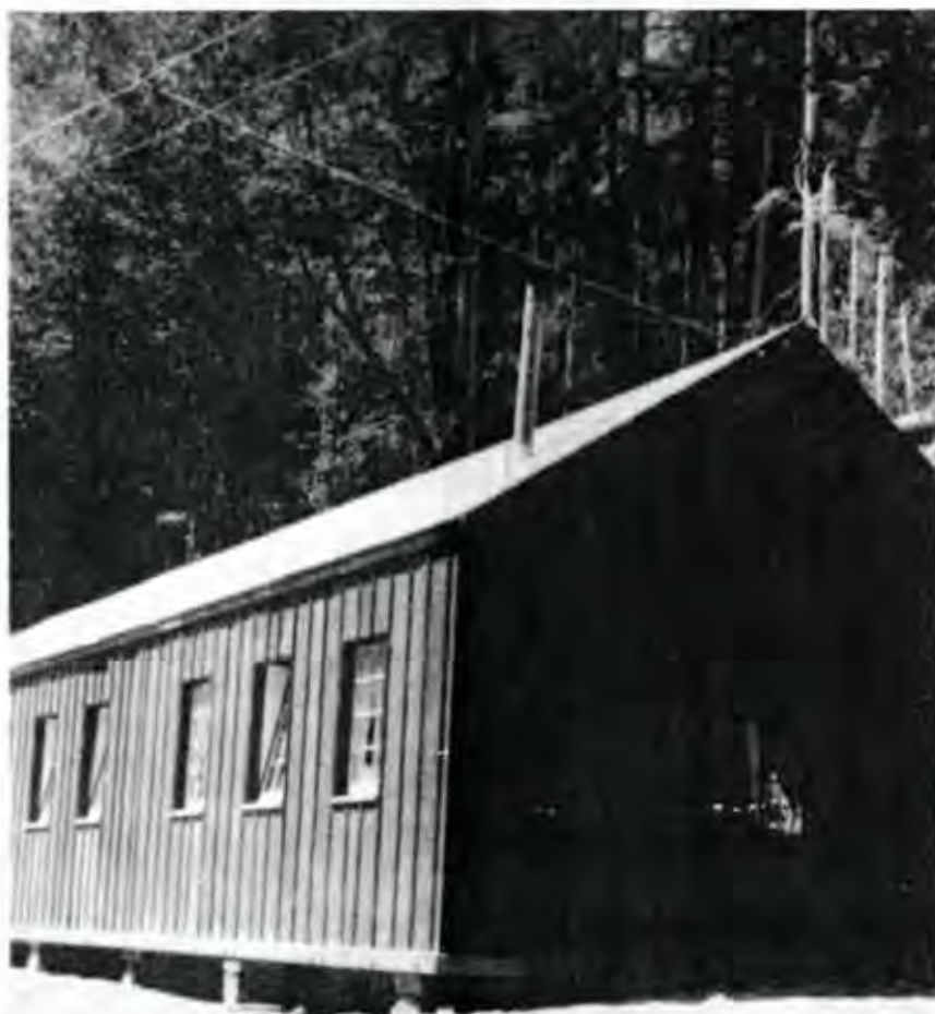
Typical CCC barracks building
