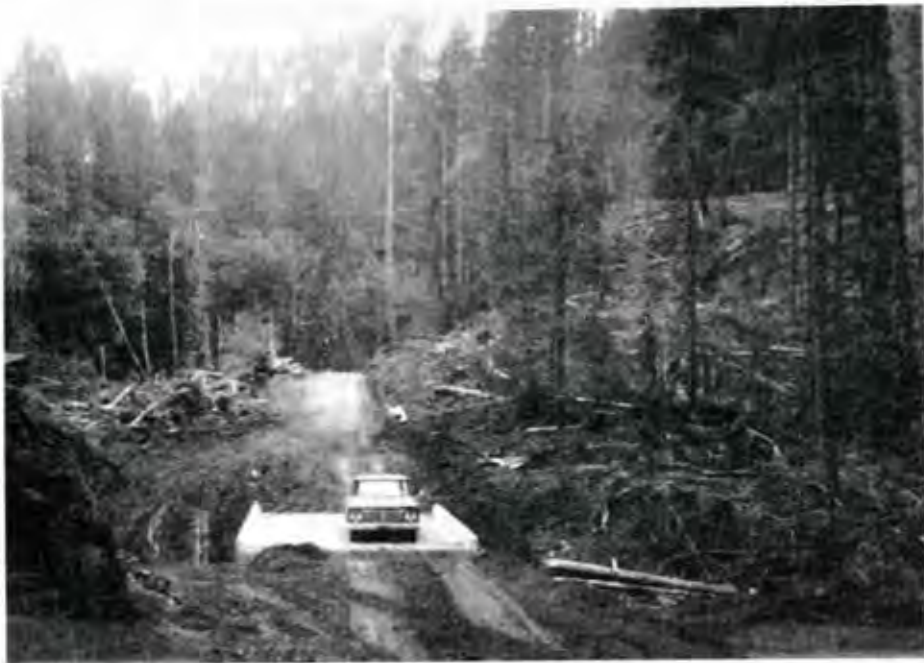
Lower Elk Creek Bridge completion, 1963. —Photo by Author.
