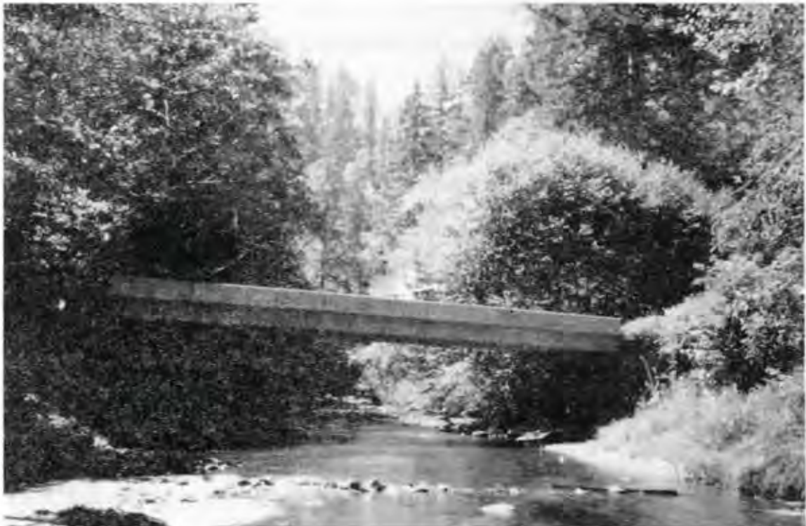
Typical concrete bridge on West Fork Millicoma. —Photo by Author.
