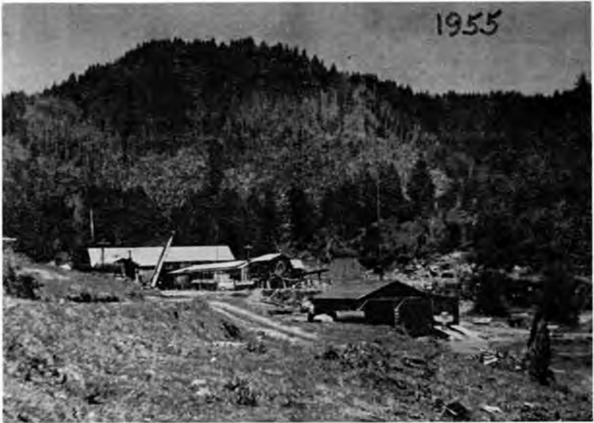
Looking north into sawmill, wigwam burner, and truck shed complex, in E \frac{1}{2} ; SE \frac{1}{4} Sec. 4, 24/11. Vaughan mill (Cooston Lumber Company) operated here in 1953, 1954, and 1955, with radio-equipped trucks hauling lumber into Coos Bay over the very narrow winding County Road. All land in this photo is today part of the Elliott Forest. The acquisition transaction did not include the twenty-seven acres to the east where the original Henry Stull (later Vaughan) home is located, although State does have a "first refusal purchase right" on that remaining acreage, in the event that property is ever sold. —Photo by author, 1955.
