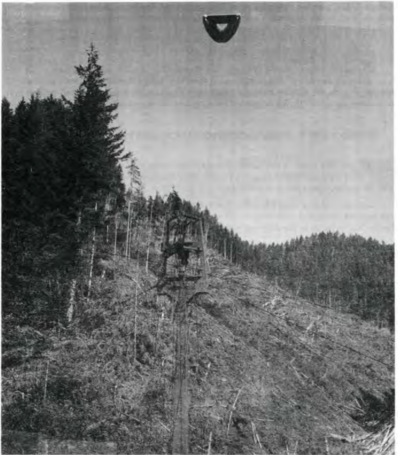
Elkside Lumber Company (Bohemia) and their experimental "V" balloon yarding the north unit of our S. Johanneson Ridge No. 1 blowdown sale. This, in 1964, was the first such operation in the State of Oregon. All yarding was downhill; here the balloon is shown moving uphill to pick up a turn. This particular balloon design was later abandoned, after technical problems. —(From my old photo files — source unknown)
