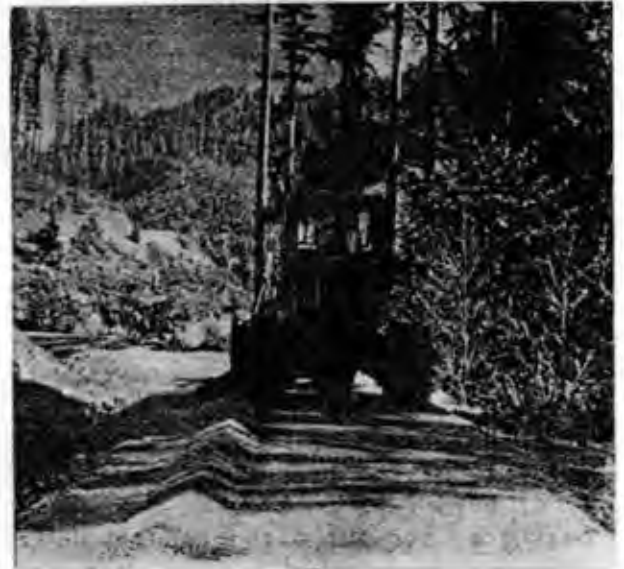
Grading on Dry Ridge
