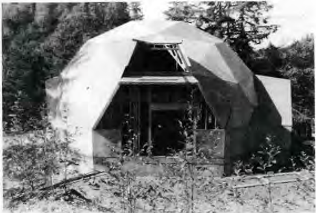
The Marlin Geodesic Dome. (2/3 complete when construction stopped in 1982).
