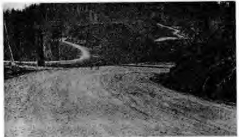
Benson Ridge Road-typical mainline
