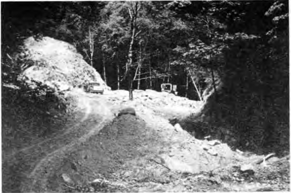
This 1958 photo shows the "channel change" project involved with construction of the Marlow Creek (Elk Ridge) mainline road (today's 1000 Road). This project was heralded as a tribute to engineering design and to environmental sensitivity, with the goal of saving Oregon taxpayers as much as $100,000 in double bridging and maintenance costs during future decades. Two similar ones were built by BLM and by Weyerhaeuser during this same time. Both Foresters and Fish Biologists were pleased by the results. —Photo by Author.
