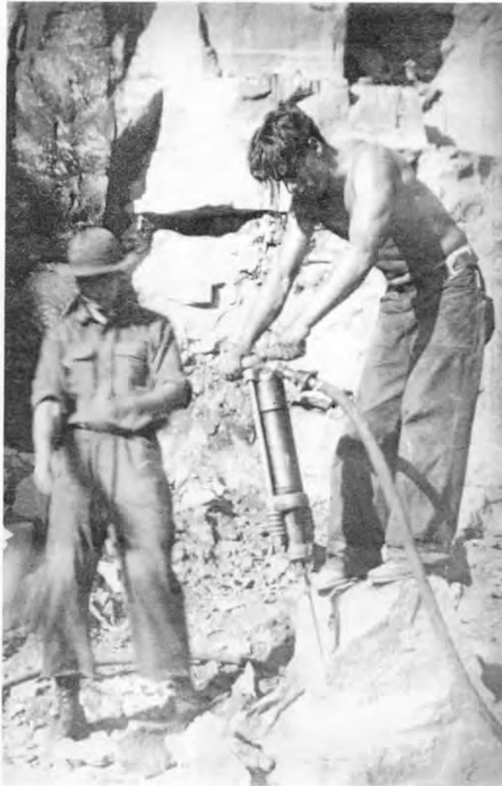
Sandstone rock drilling and blasting was a major activity during the construction of the Scholfield-Umpcoos Ridge Roads. Hardhats were unknown, but some wore "pith helmets" such as this man has. Surprisingly, injuries were uncommon. —Photo courtesy C.F.P.A. files
