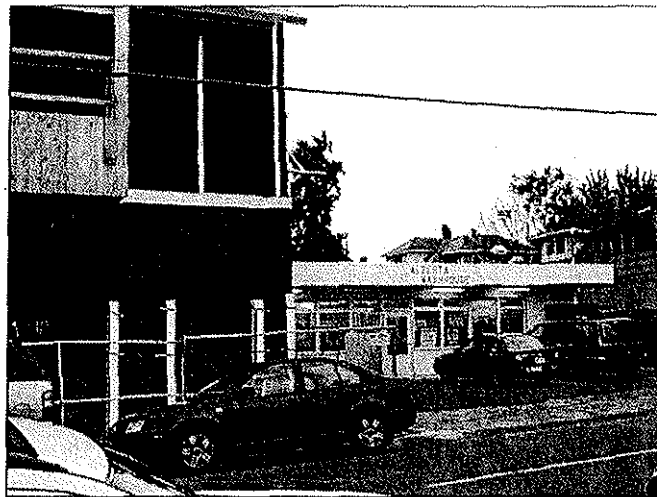
Figure 2: Construction of a new office building next to the Alberta Washhouse at NE 22 nd and Alberta.
