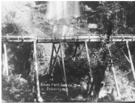
Silver Creek Bridge at base of Silver Falls, 1913. The two bents at fall right were rotten and collapsed with a load of lumber in 1941.
