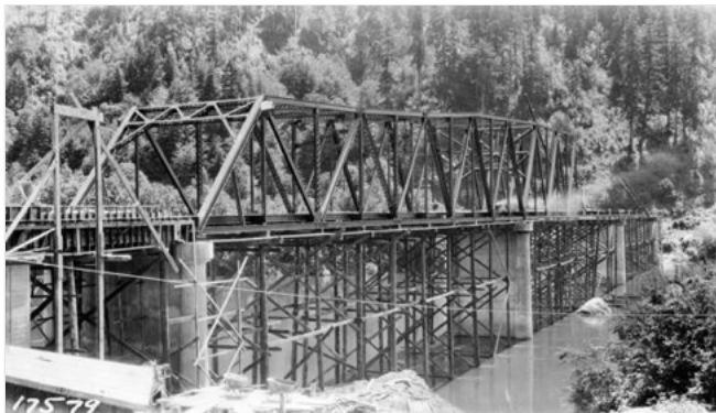
Several South Coast bridges also designed by McCullough
