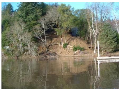
**Figure 4.5. Surface erosion in a construction site. North Lake.**
