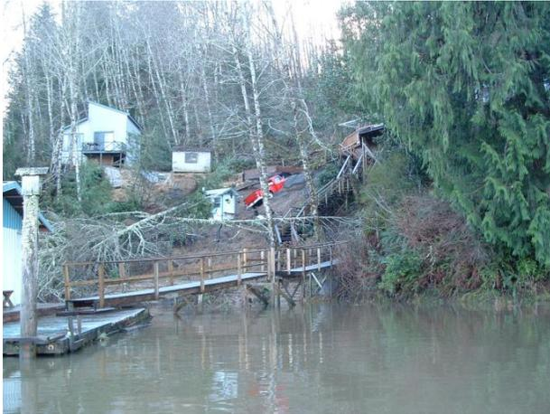
Figure 4.6 shows the effects of placing a septic system on a very steep slope. Not evident in the photo is the approximately 50% slope above the home. When a late December storm dumped eight inches of rain in thirty-six hours, the already saturated soil in the drain field gave way.
