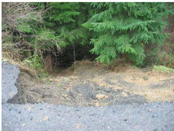
**Figure 4.11. Road related landslide, moving downstream.**
